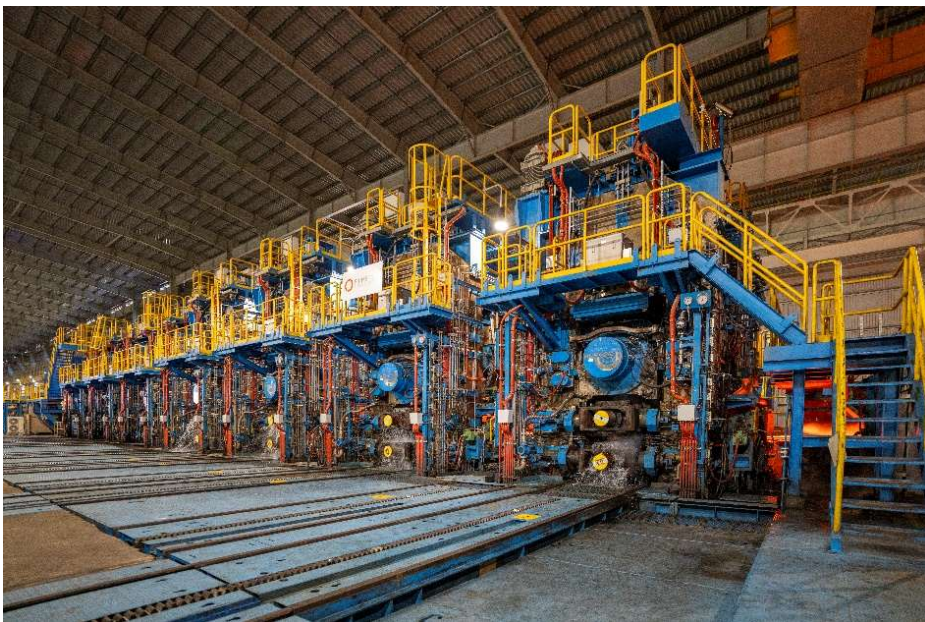
The hot-strip mill from Primetals Technologies with a rated capacity of 5.5 million tons per year.
